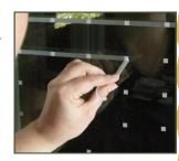
For vertical striping, the stripes should be placed a maximum of 10.00 cm (4.00 in) apart.
