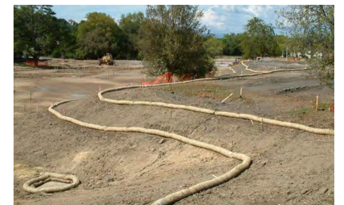
Erosion control at development site
