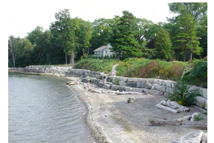
Shoreline protection structure coordinated among landowners
