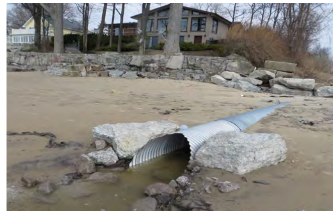
Bernard Beach Storm Sewer
