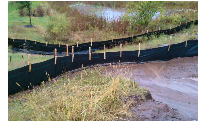
Erosion control fencing
