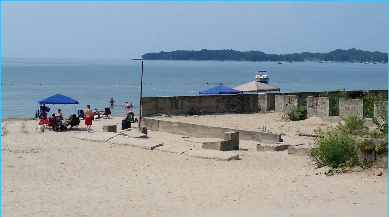
Remnant building foundations at Bay Beach
